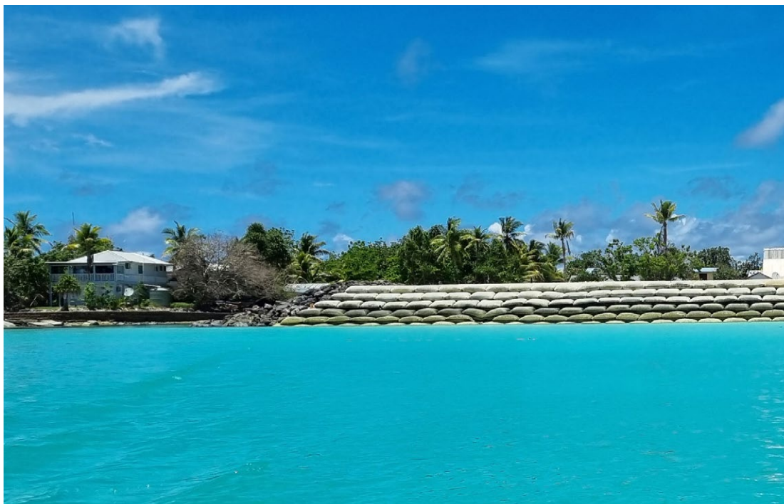
A land reclamation project in Funafuti, predicted to last for approximately 25 years, where sand is dredged from the lagoon and placed in large bags that settle for up to a year before seedlings are planted, then eventually buildings will be constructed and people can move onto the new land. © Amnesty International
