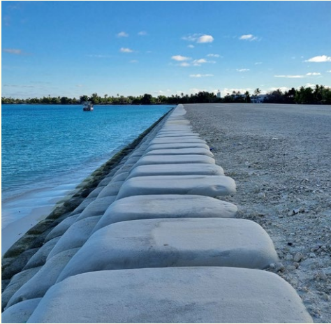
A land reclamation project in Funafuti, predicted to last for approximately 25 years, where sand is dredged from the lagoon and placed in large bags that settle for up to a year before seedlings are planted, then eventually buildings will be constructed and people can move onto the new land. © Amnesty International
