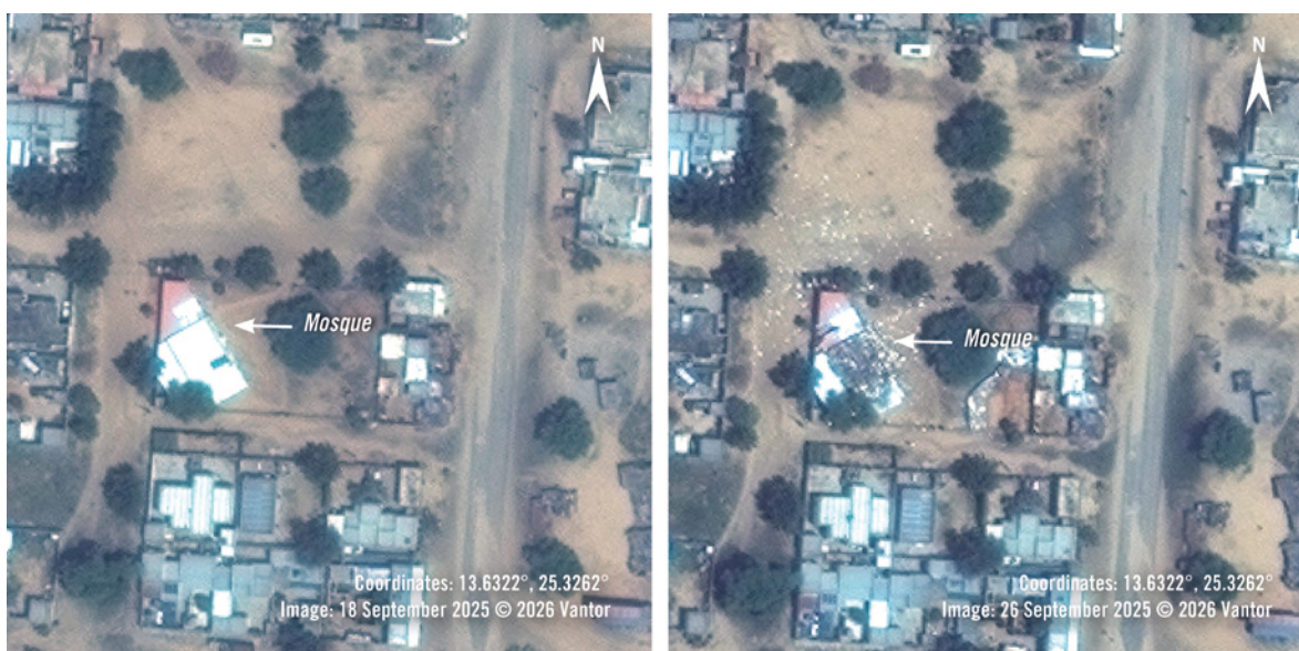
© ↑ Satellite imagery from 18 September shows El Safiya mosque. On 26 September, satellite imagery shows major destruction at the mosque.
