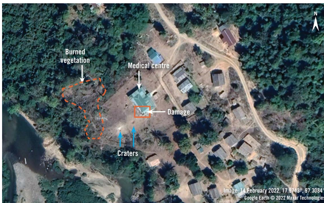
Satellite imagery from 14 February 2022 shows a health centre in Wah Ka Der, Kayin State. Two craters are visible as is damage on the health centre's southwest corner. Low resolution imagery (not shown) confirms the vegetation was burned between 2-7 January 2022 and at least one crater first appeared between 11-17 January 2022.
