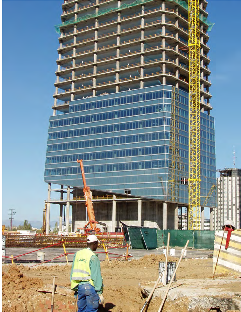
Sport City Towers construction. Madrid. © Cristina Arias/Cover/Getty Images.
