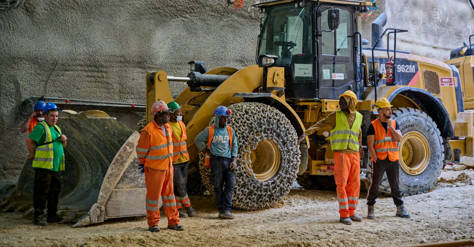
Workers stand in front of large machinery as they wait for the wall to be breached at the future Estrela underground station on May 28, 2022 in Lisbon, Portugal. © Horacio Villalobos/Corbis via Getty Images
